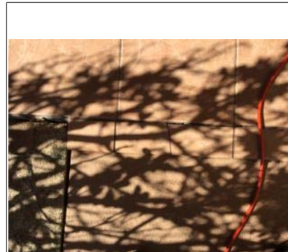
Cracked front porch floor tile
